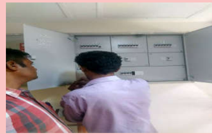
Energy Audit at M/s.TEMPLE CITY Madurai
